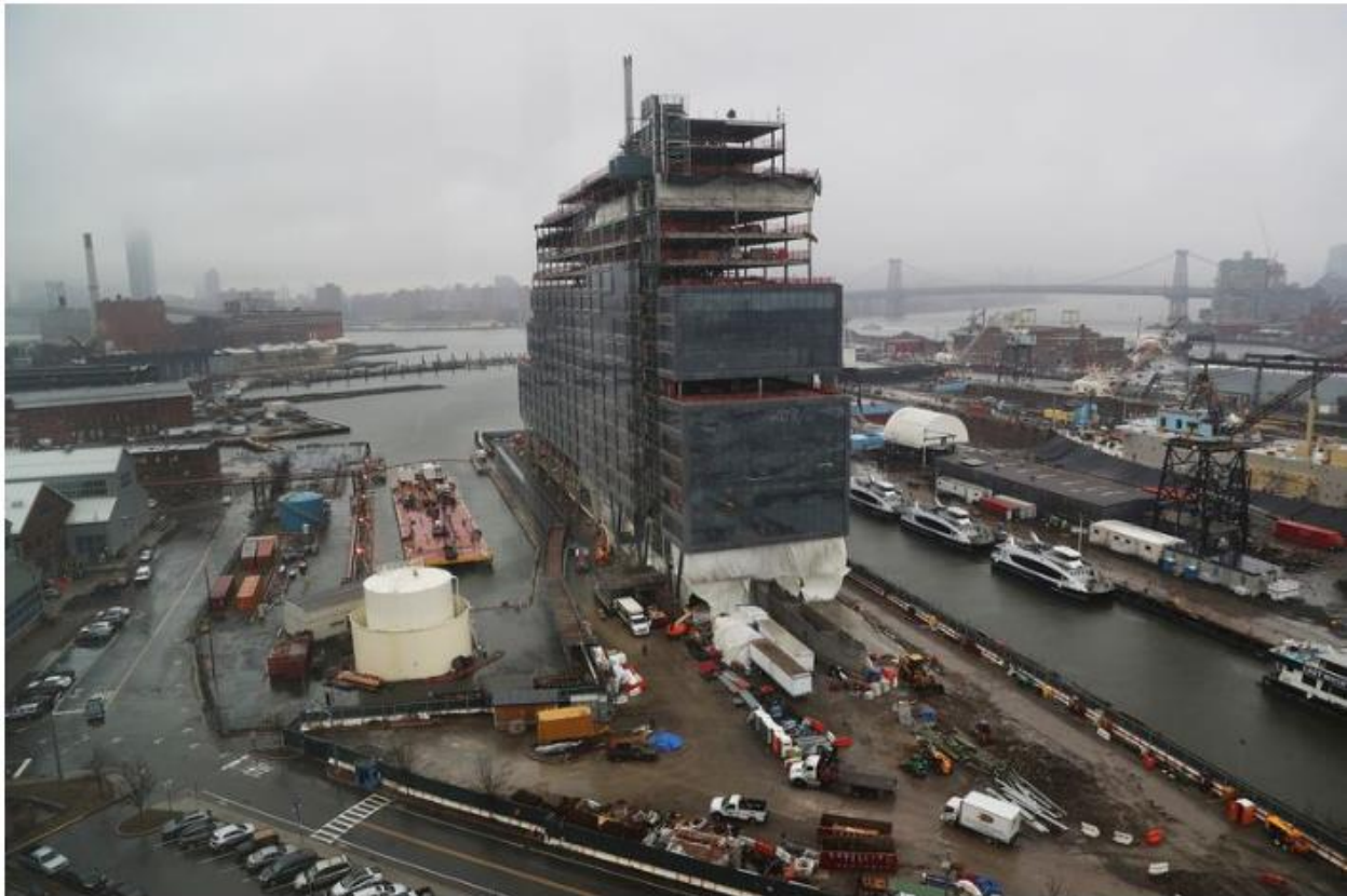
Construction on Dock 72 at the Brooklyn Navy Yard. Photographer: Victor J. Blue/Bloomberg
